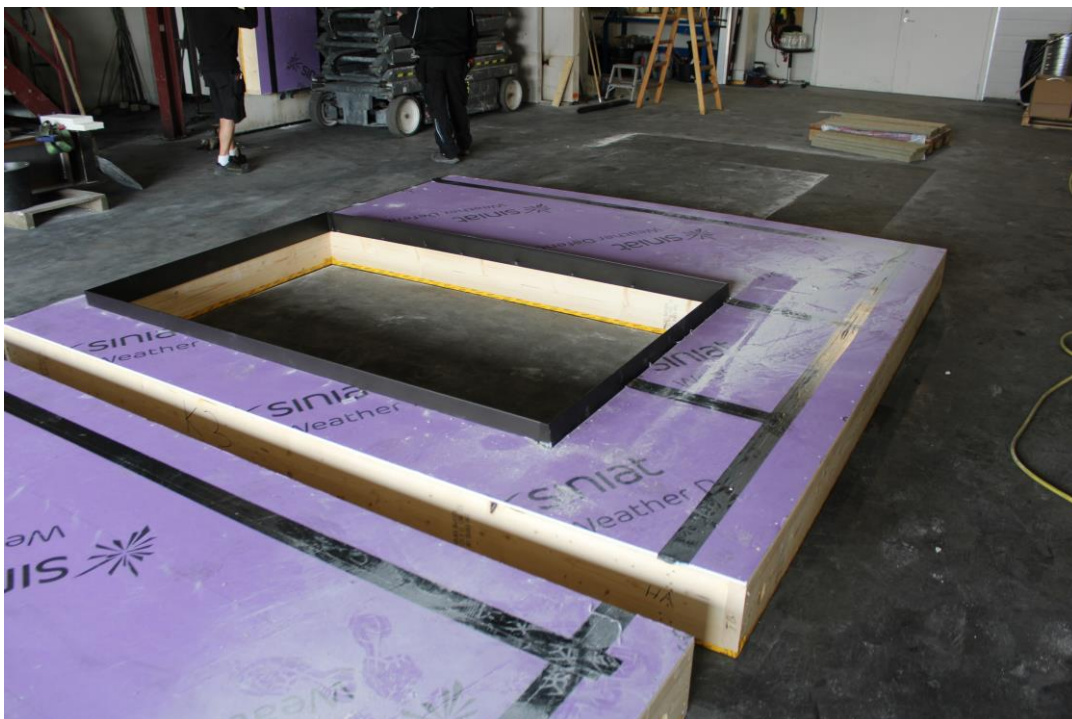
Photo No. 2 Flashing added around the windows and fire chamber.
