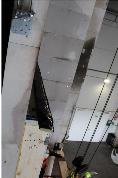
Photo No. 5 Tight insulation placed between the prefabricated elements
