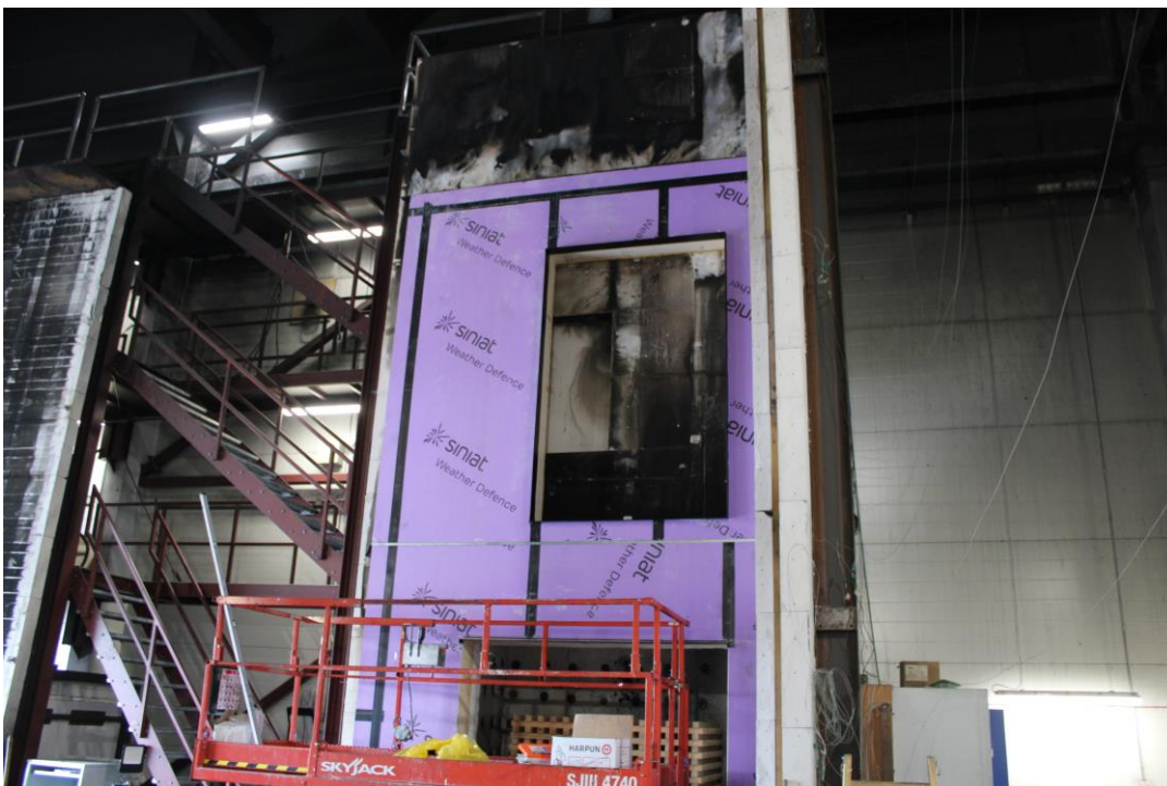
Photo No. 4 Fixing of prefabricated elements.
