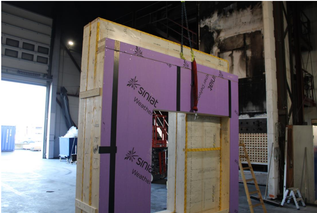
Photo No. 1 Prefabricated elements before mounted to the façade rig.
