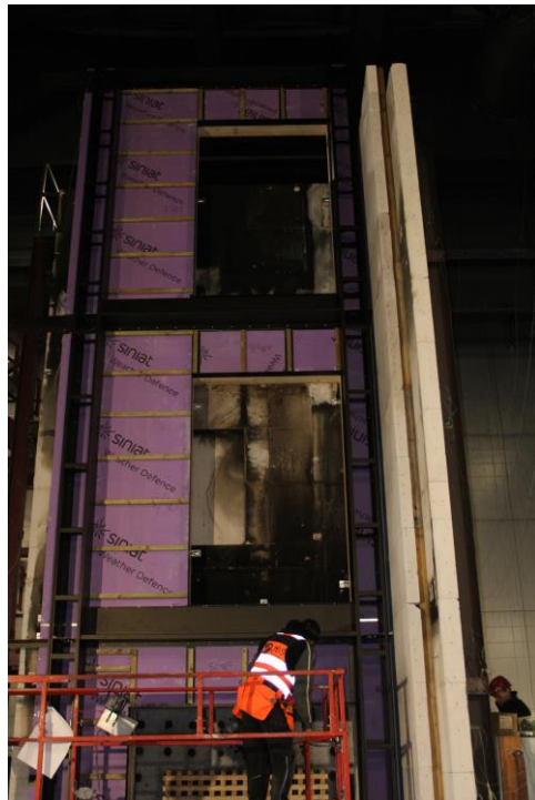
Photo No. 8 Horizontal and vertical formworks have been mounted.
